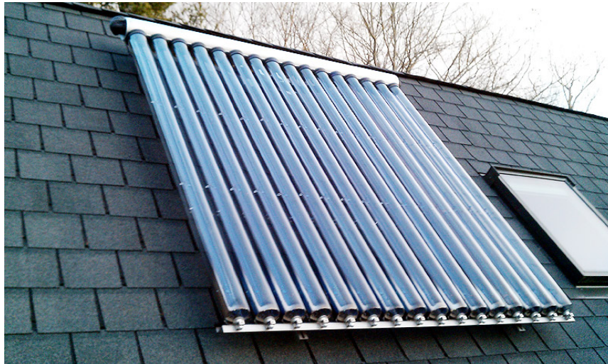
Figure 10.13: A rooftop solar thermal array for domestic water heating.
