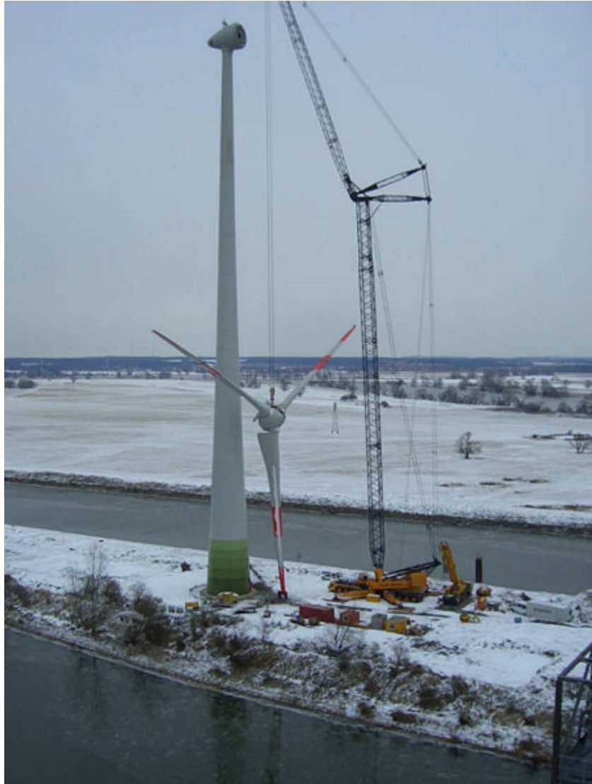
Figure 5: Erection of an Enercon E70-4 in Germany
