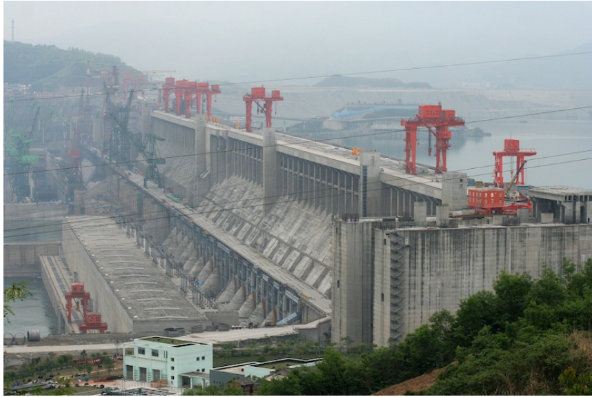
Figure 3.11: Construction of the Three Gorges Dam (2006).
