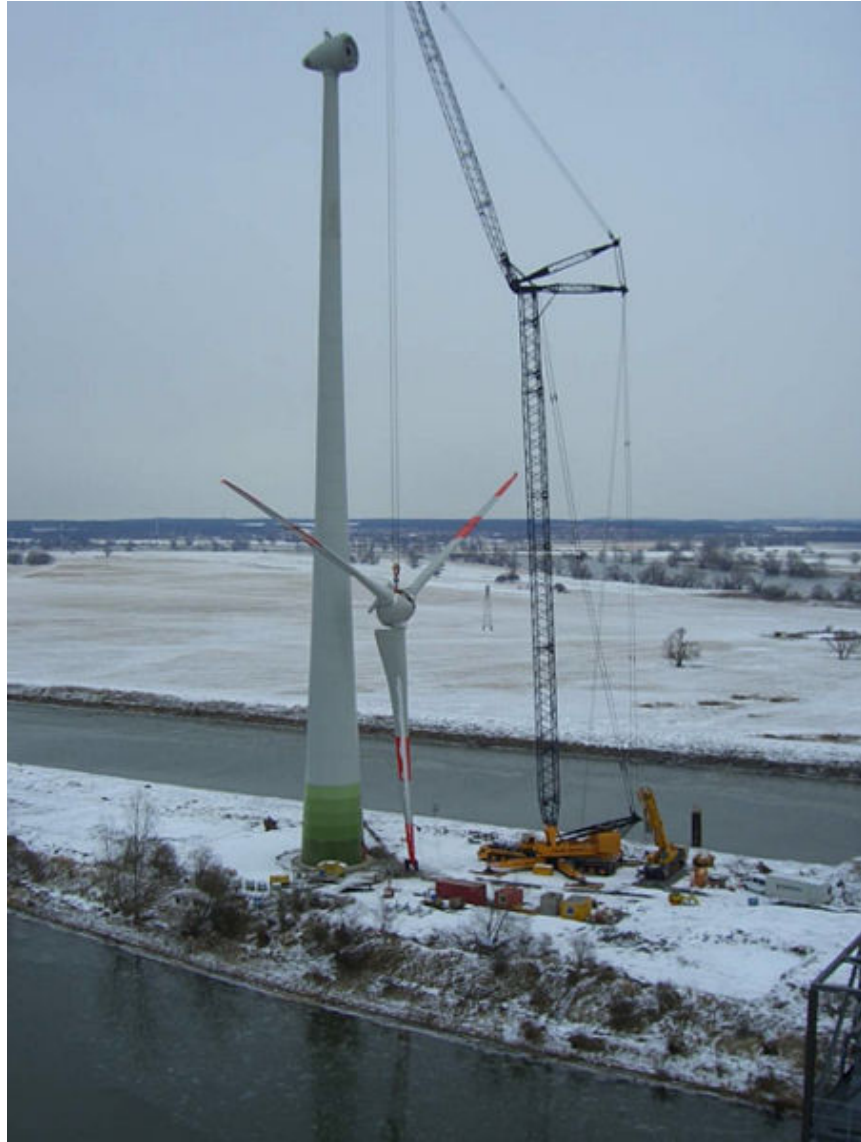
Figure 3.9: Erection of an Enercon E70-4 in Germany
