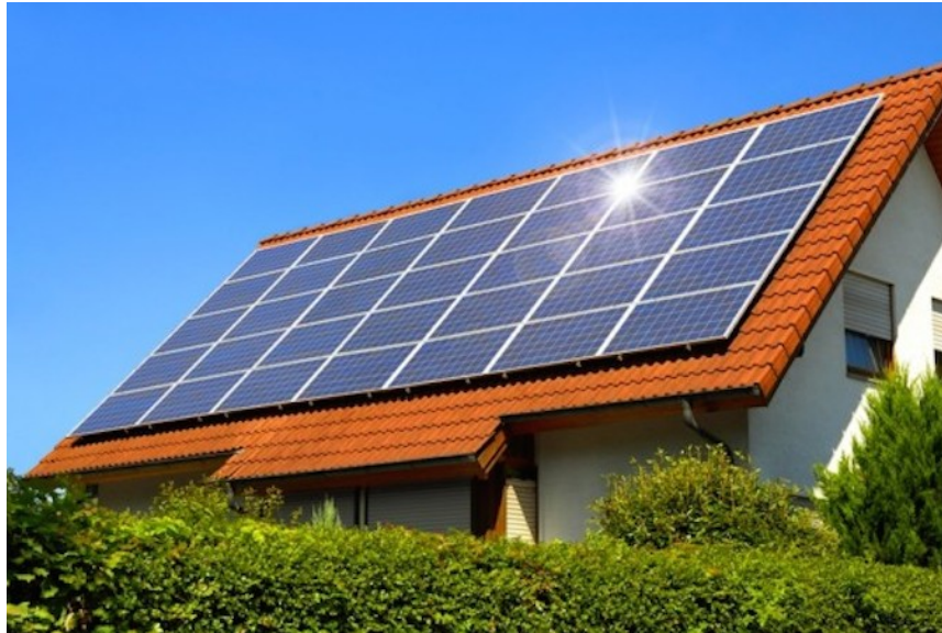
Figure 2.1: A rooftop array of photovoltaic cells.
