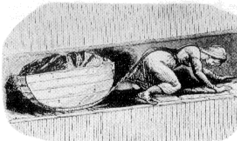
Figure 6.3: A girl pulling a coaltub through the narrow space left by removal of coal from a seam. (Public domain)
