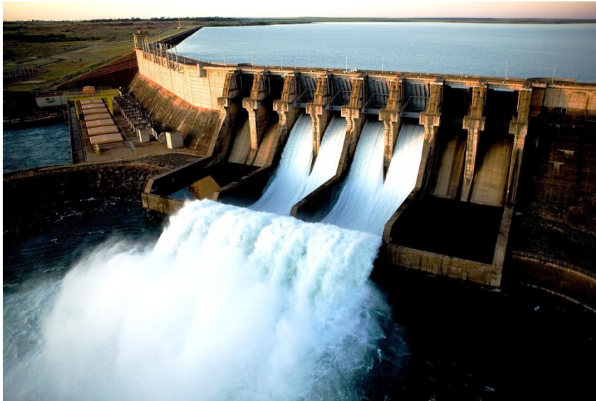
Figure 3.17: Hydroelectric power does not suffer from the problem of intermittency, but may sometimes produce undesirable social and ecological impacts.
