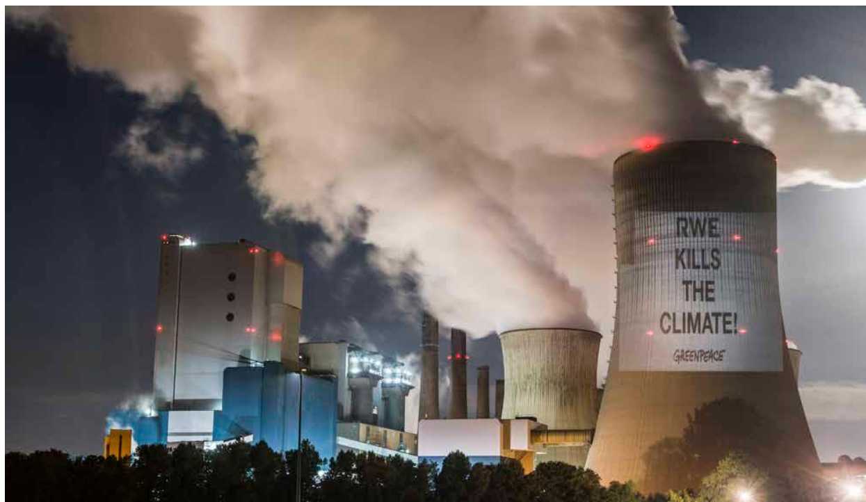
Figure 3.6: A coal-fired power plant.
