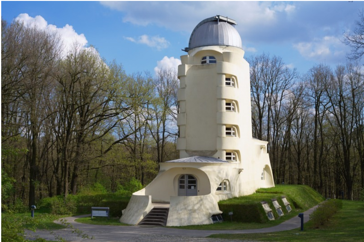
Fig. 12.5.1. The Einstein Tower (1924) is an astrophysical observatory and also a masterpiece of the history of German architecture designed by Erich Mendelsohn (1857-1953). Photograph © R. Arlt.
