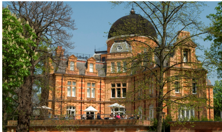
Fig. 12.1.2. Top: The Meridian Building in the 1930s, before the 1960s reconstruction work. Middle: The Meridian Building and the Great Equatorial Building, 2009. Bottom: The South Building, 2009. Photographs © National Maritime Museum
