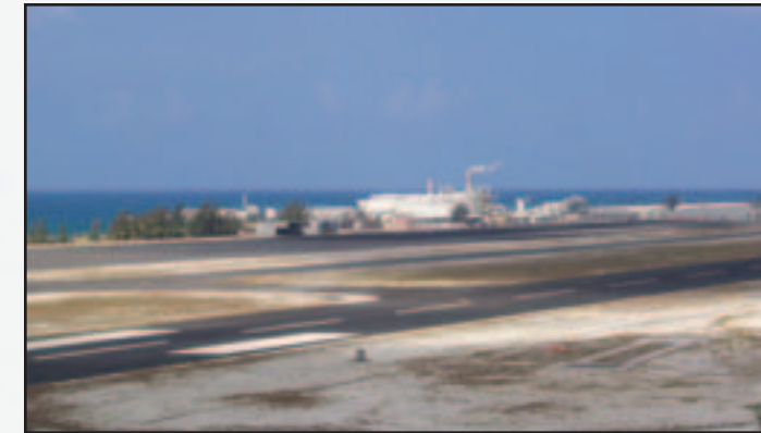
Johnston Atoll Chemical Agent Disposal System (JACADS) plant from across runway.
