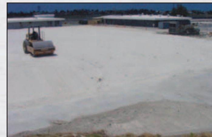
Creating a coral cap over the former site of the Munitions Demilitarization Building (MDB).
