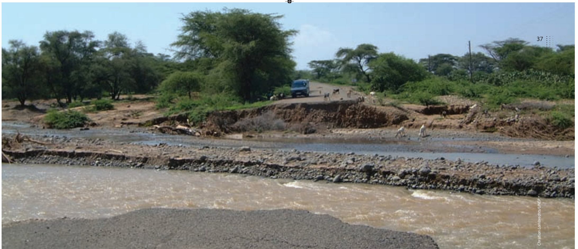
Flash floods wash out a section of a road in Baringo District
