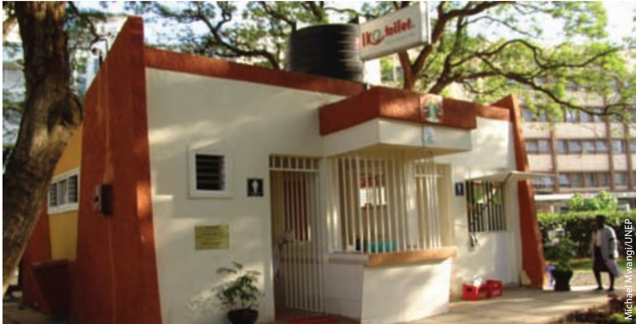
The City Council of Nairobi improving access to better sanitation facilities by constructing more facilities within common areas
