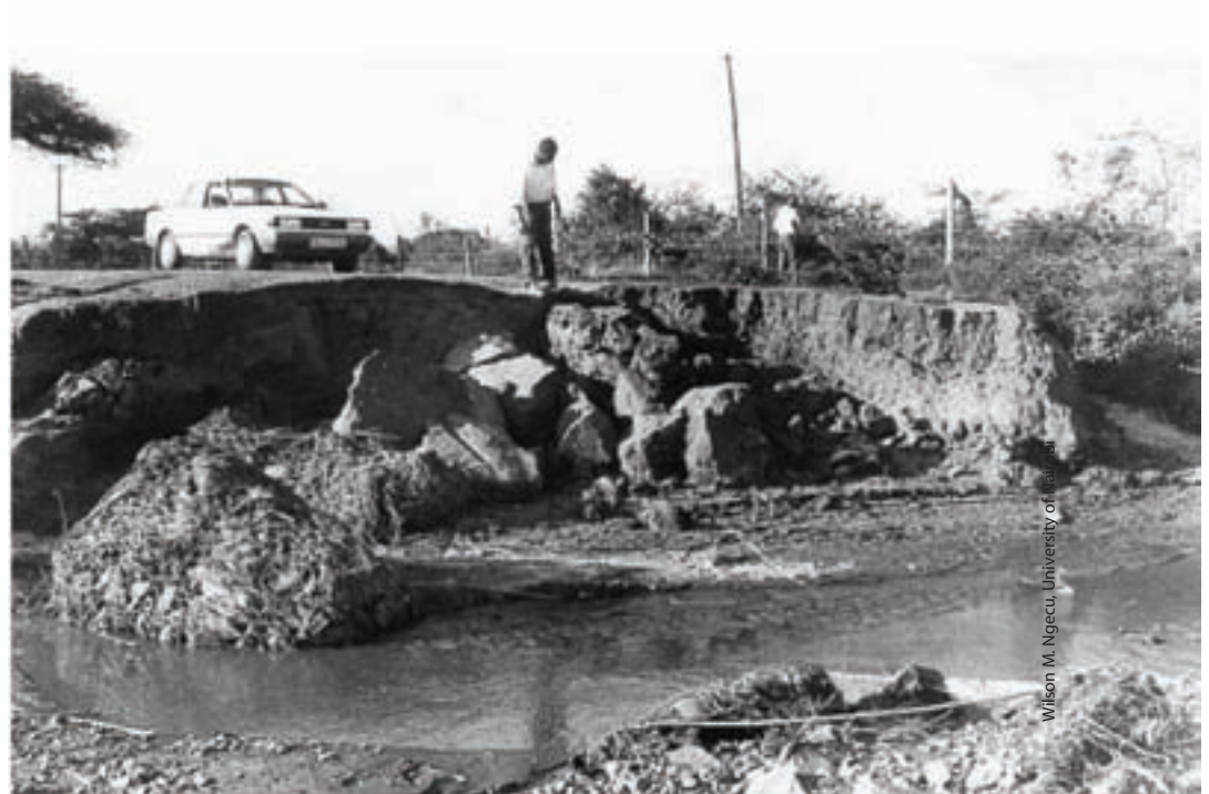
A section of Massii-Makueni high were a major bridge was destroyed by a late 1990s landslide
