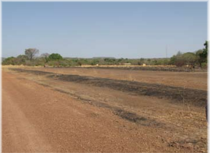
The airport runway in the village of Falea
