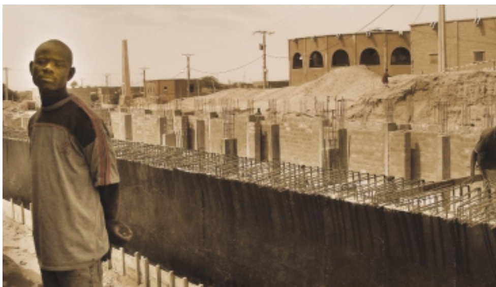
The new Ahmed Baba library building under construction.
