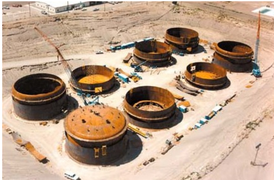
Hanford Tanks Under Construction (Department of Energy photo)
