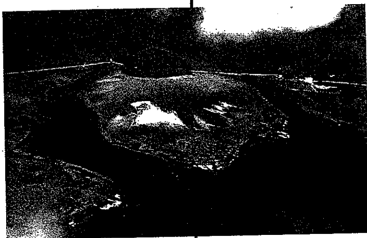
Causeways connecting the islands are vital to local transportation and economic activity. They are at risk from sea level rise and storm damage as climate change
